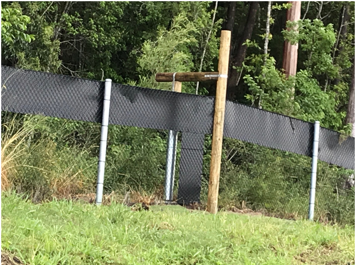
Figure 3. Koala escape pole along Wilson Road
