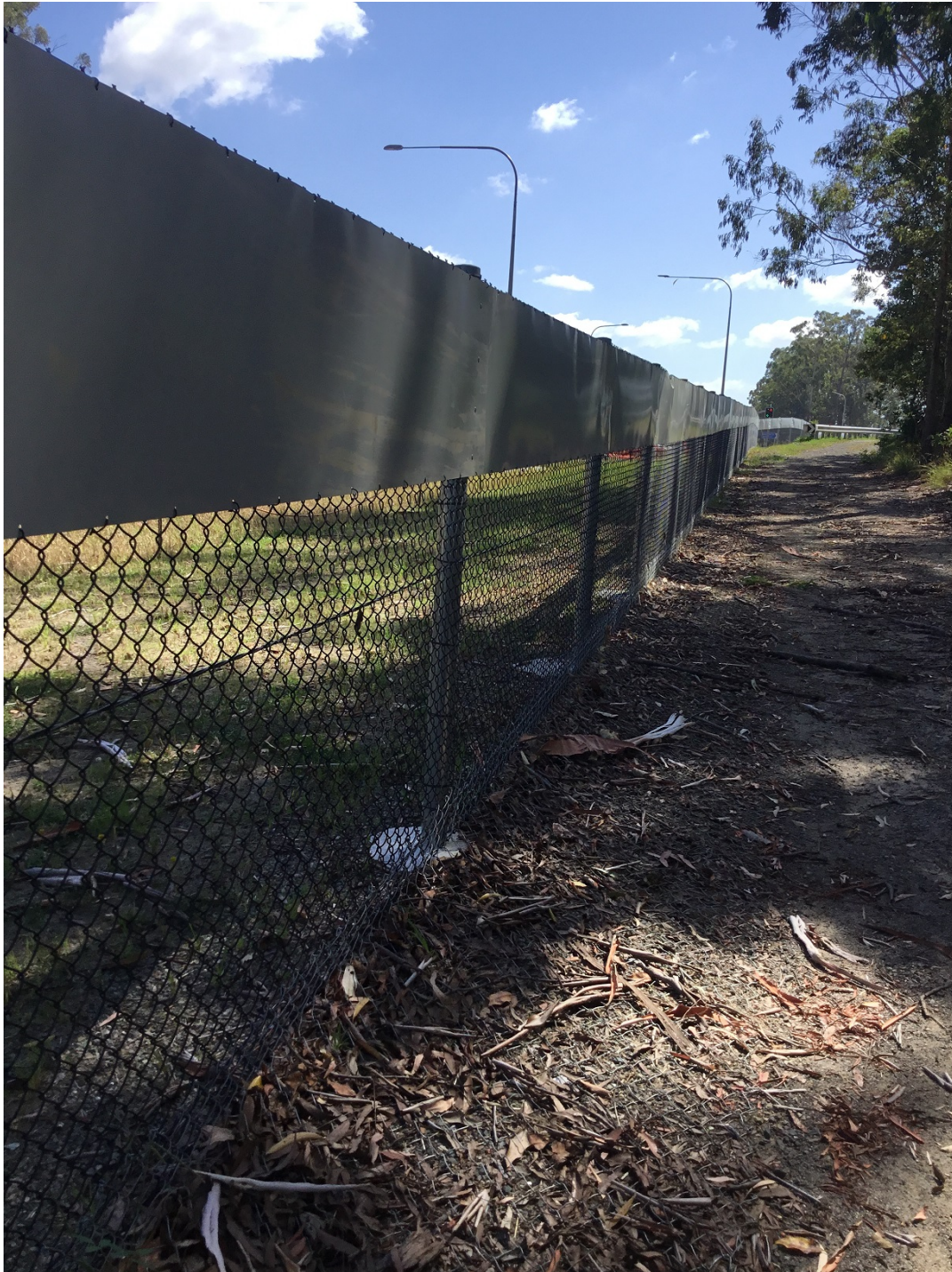
Figure 1. Permanent fauna fence adjacent to Mooloolah Cemetery
