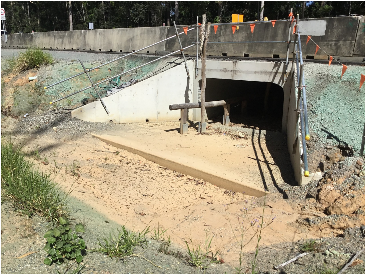
Figure 2. Steve Irwin Way fauna crossing (in progress)
