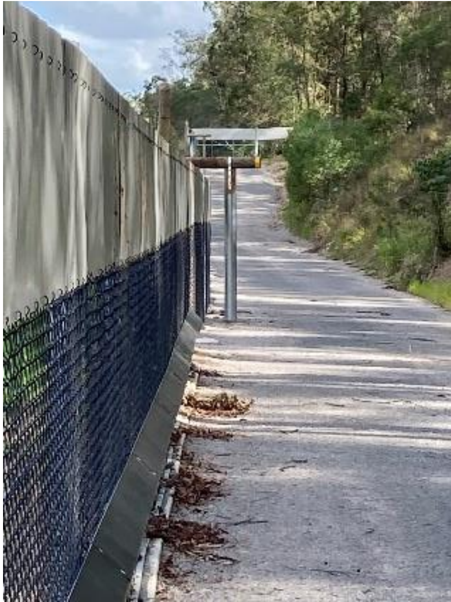
Figure 1. Permanent fauna fence with frog exclusion fencing and Koala escape pole adjacent to Bruce Highway
