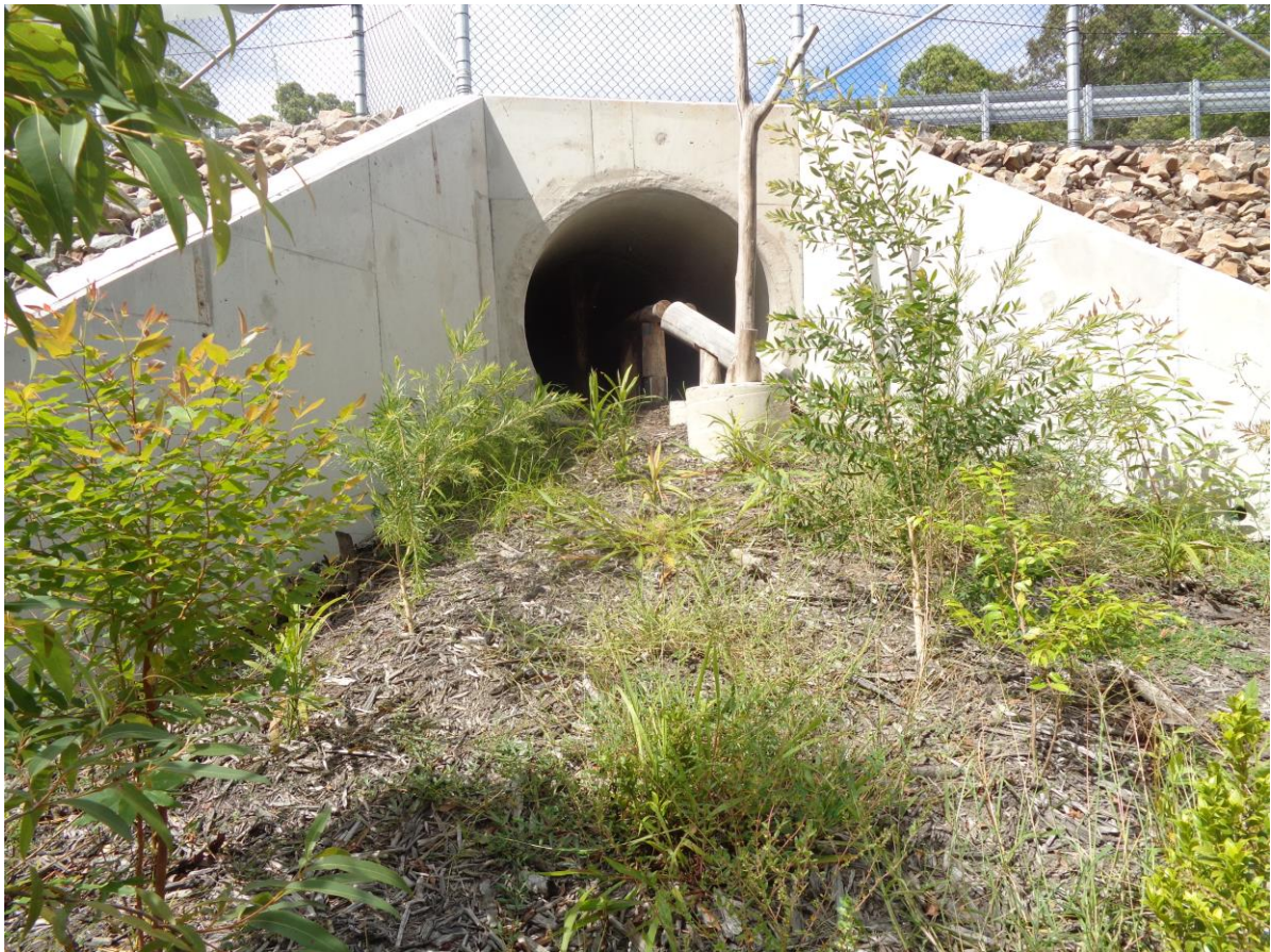
Figure 5. Completed Northern Fauna passage
