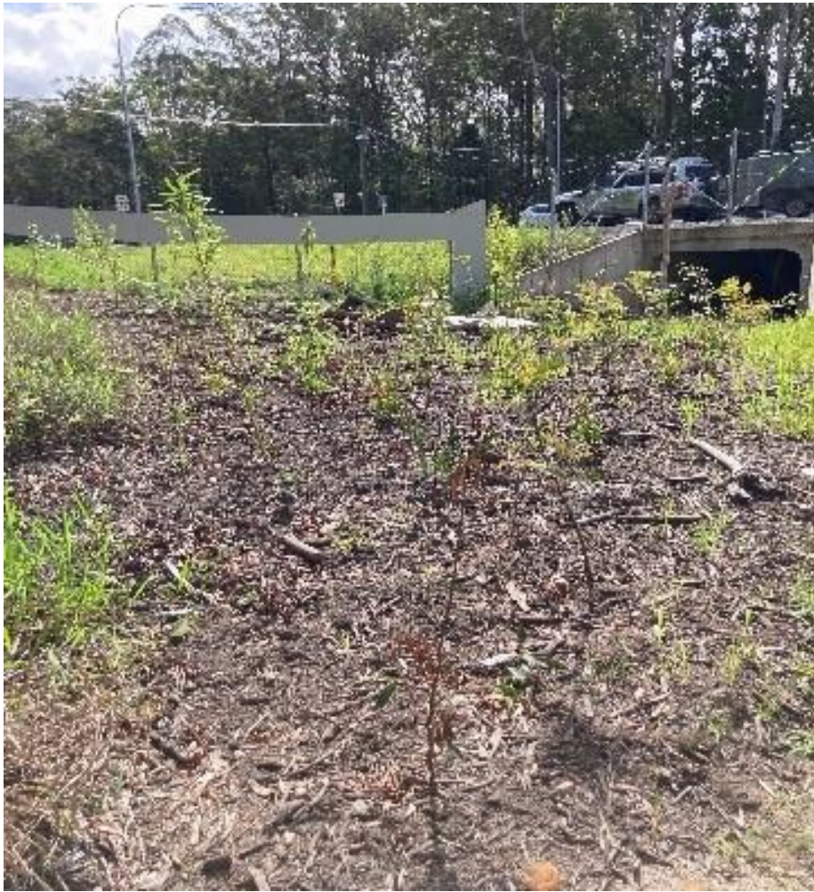
Figure 2. Completed Steve Irwin Way Fauna passage
