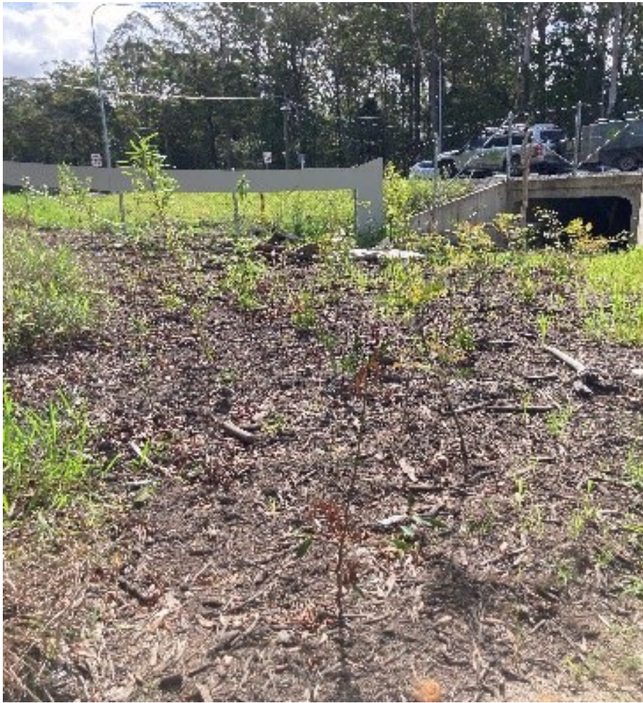
Figure 2. Completed Steve Irwin Way fauna passage
