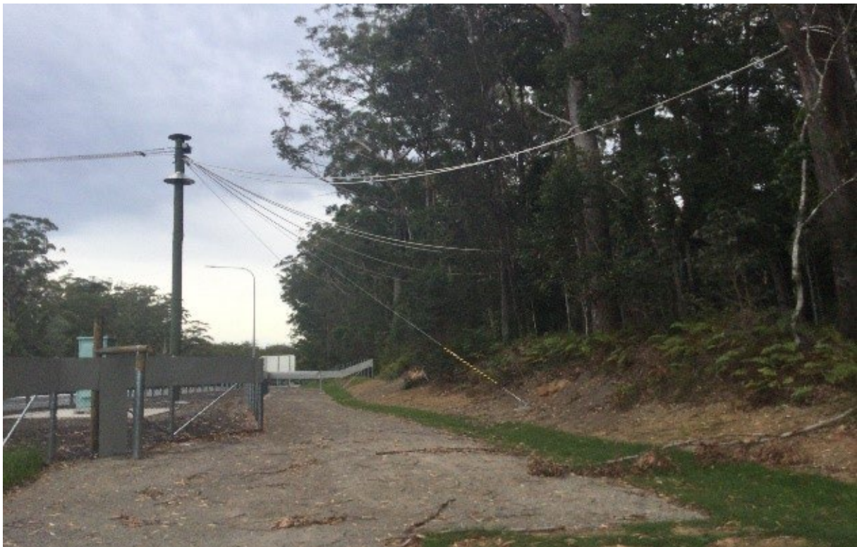
Figure 11. Rope bridge across Steve Irwin Way
