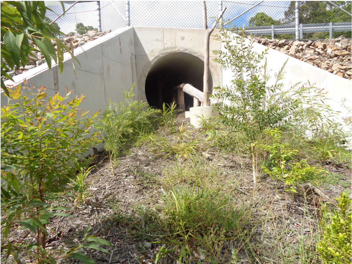
Figure 5. Completed northern fauna passage
