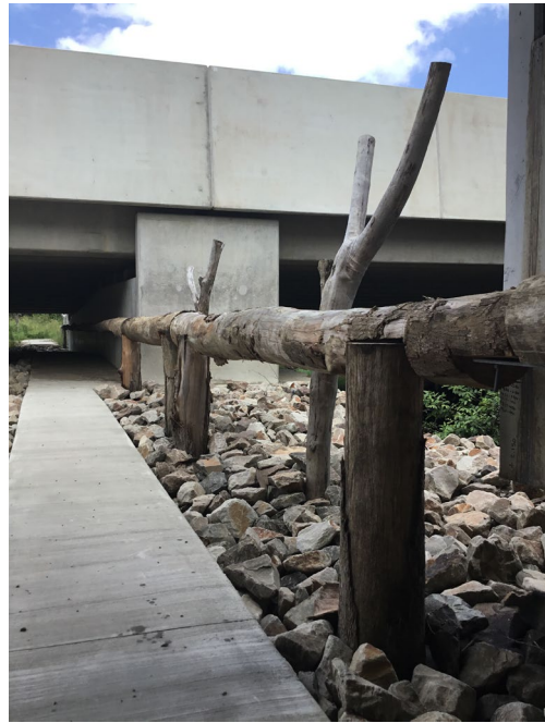
Figure 9 and 10. Fauna structures installed at Mooloolah River
