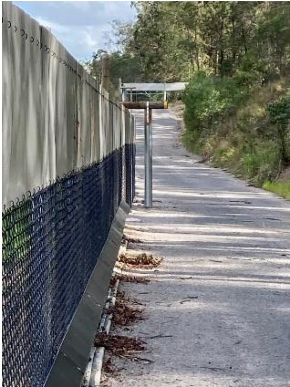
Photo Plate 1. Permanent fauna fence with frog exclusion fencing and Koala escape pole adjacent to Bruce Highway
