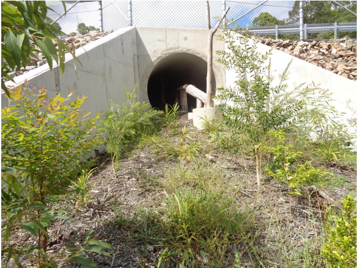
Photo Plate 5. Completed northern fauna passage
