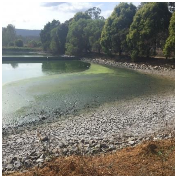
Figure A-4 Dewatered Urban Utilities lagoon prior to biosolids removal (Urban Utilities, 2021)
