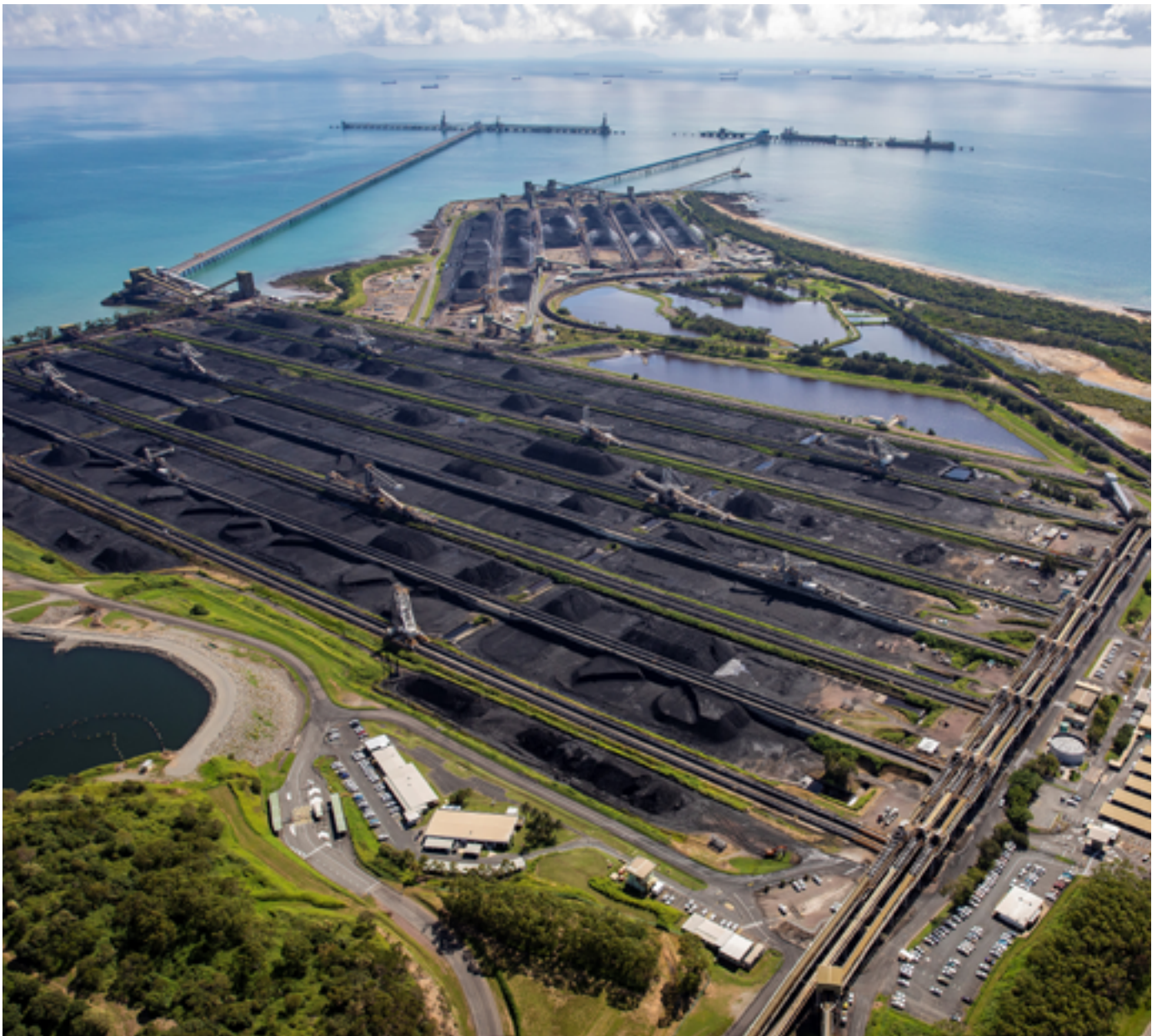
Coal stockpiles at the Port of Hay Point. Source: NQBP
