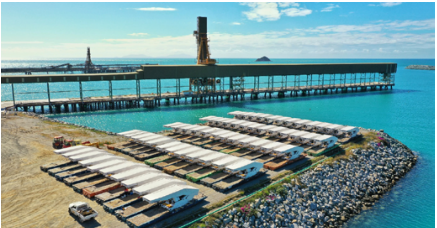
Laydown area with cargo - Port of Mackay. Source: NQBP
