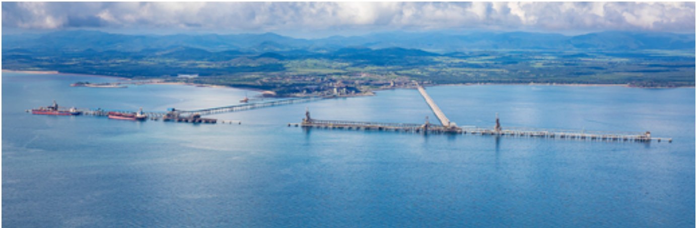
Aerial view - Port of Hay Point. Source: NQBP
