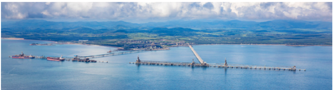
Aerial view - Port of Hay Point. Source: NQBP
