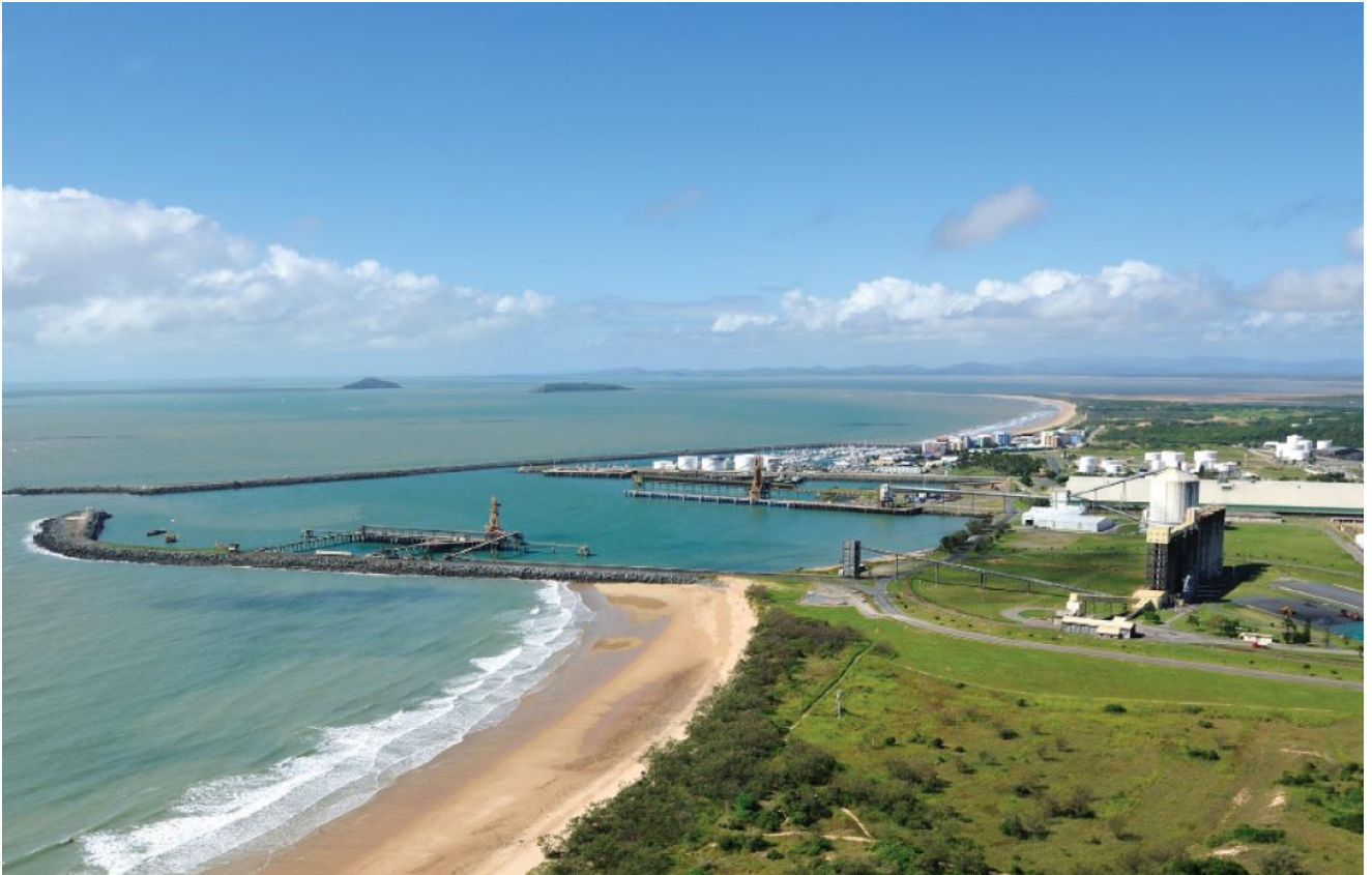
Figure 36: View south from Slade Point Nature Reserve towards the Port of Mackay
