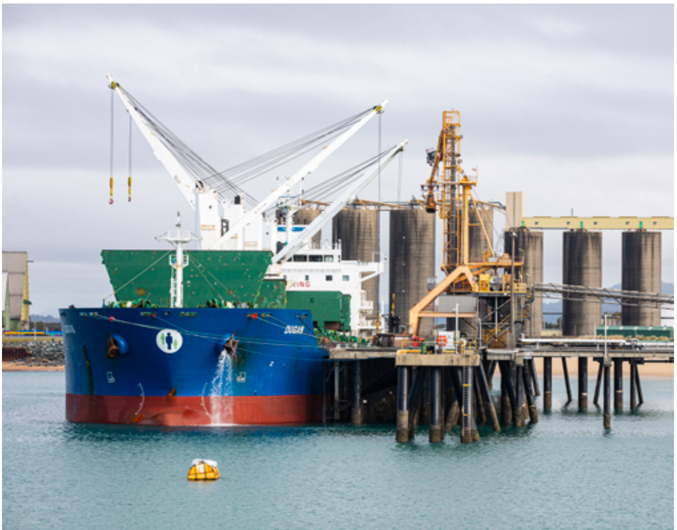
Ship loading at the Port of Mackay – Wharf 5. Source: NQBP
