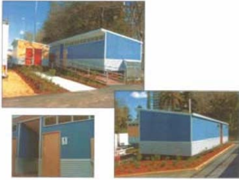
Use of different colours and materials, eaves and wooden slats as skirting to hide building services.
