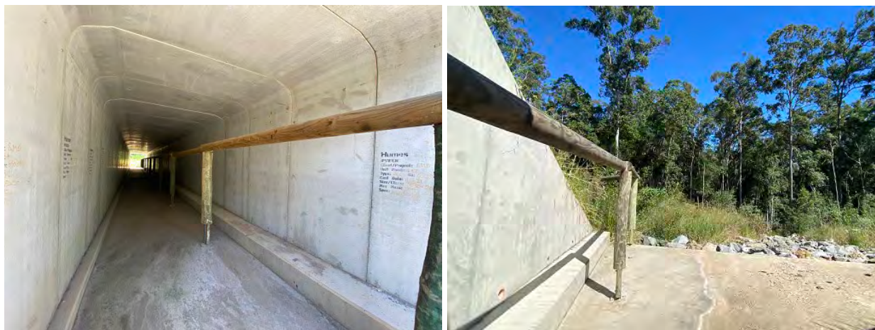
Plate 4.2 Koala crossing beneath the project
