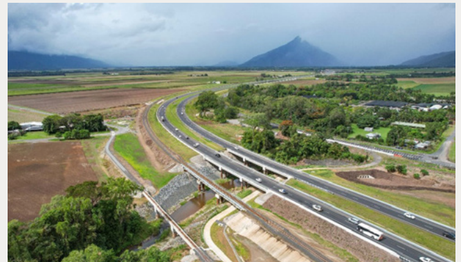
The John Davies Bridge built as part of the Bruce Highway, Cairns Southern Access Corridor (Stage 3), E2G project. Source: TMR.
