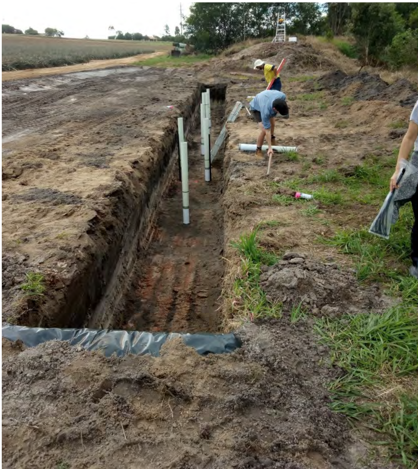
Figure 10: Groundwater monitoring piezometers installed to monitor groundwater flow through a bioreactor wall.
