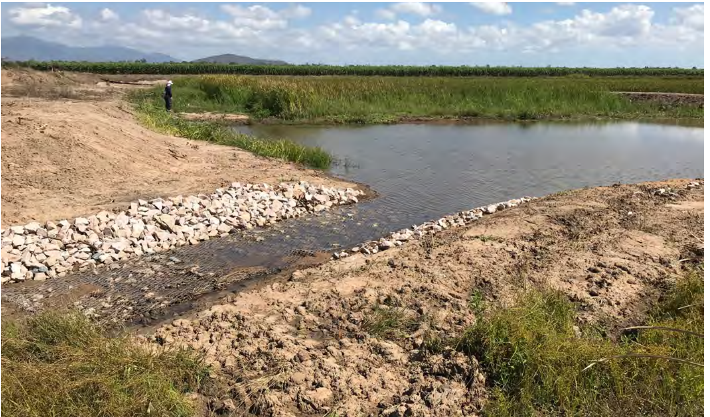
Figure 8: Drain forming the inlet to a treatment wetland.
