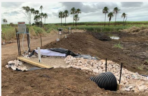
Figure 3 Completed bioreactor showing inlet structure with pipe from upslope cane block directing water into the inlet pit filled with washed river gravel (left). Excess flow bypasses the structure to a low-lying area on the right.
