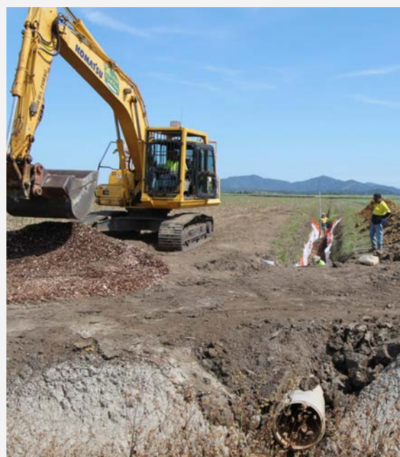
Figure 1 Construction of the in-line bioreactor bed within an agricultural drain.
