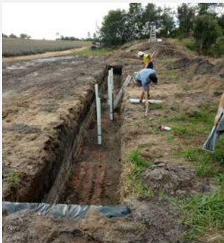
Figure 2 Construction of bioreactor walls.
