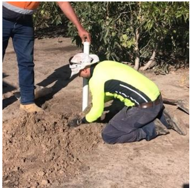
Figure 4: Backfill the rest of the hole with soil and compact it.
