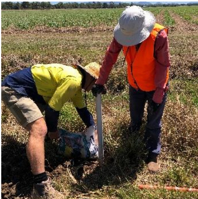
Figure 2: Install the piezometer in the hole.
