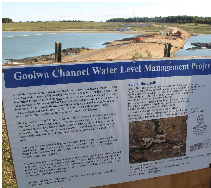
Figure A62-8: The main temporary flow regulator across the Goolwa Channel
