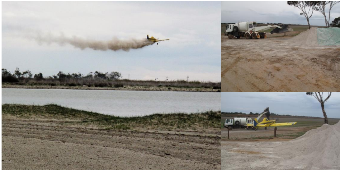
Figure A62-7: Aerial application of limestone in Boggy Lake, SA
