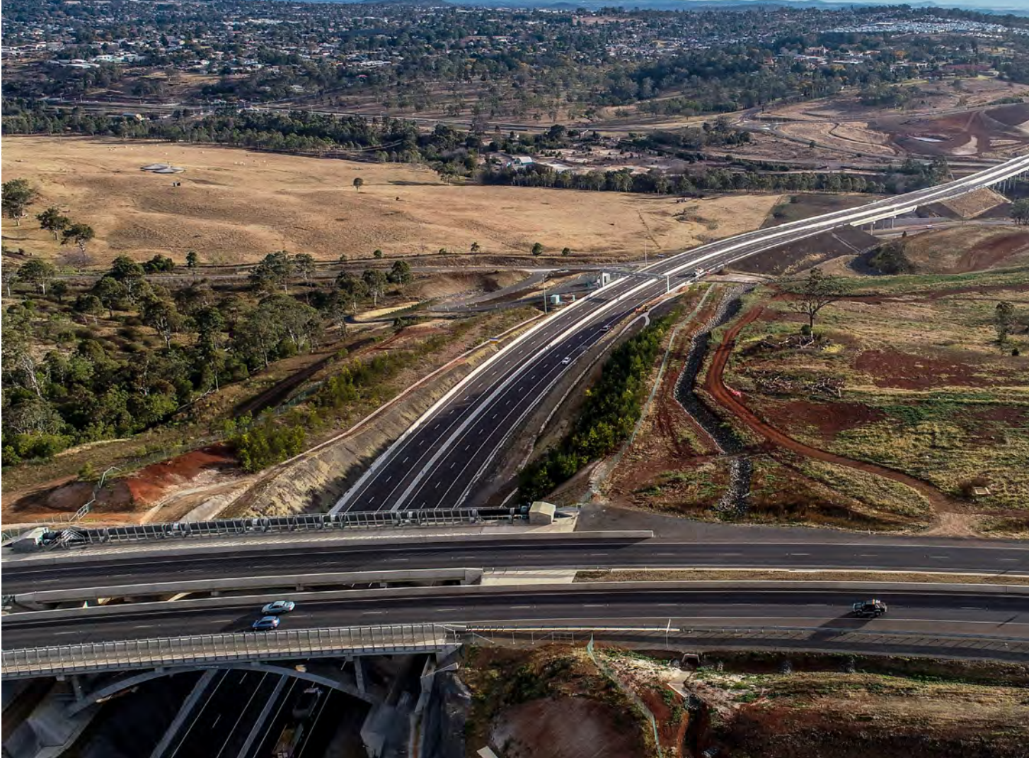
Aerial view of the Toowoomba Second Range Crossing.
