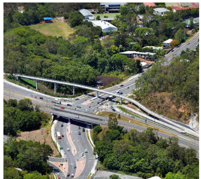
Moggill Road Cycle Bridge adjacent the Western Freeway in Indooroopilly, Brisbane.
