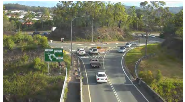
The upgraded Exit 49 on the M1 at Pimpama, including installation of roundabout metering traffic signals.
