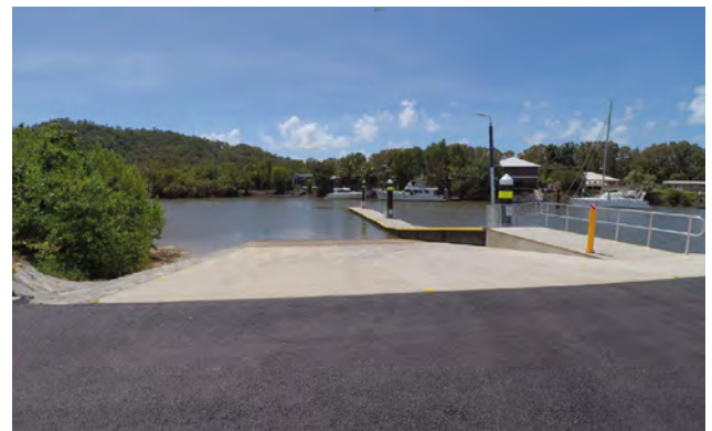
Reconstructed two-lane boat ramp at the Bluewater Marina in Cairns.
