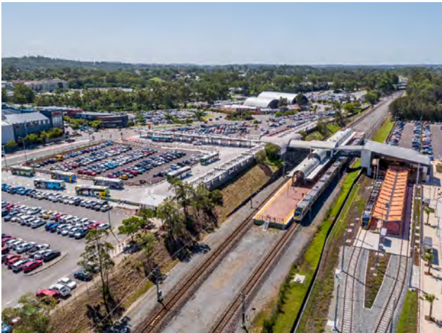
Helensvale station: New multi-modal interchange enabling seamless customer transfers between trams, trains and buses at Helensvale (Photo credit: MultiModal drones).
