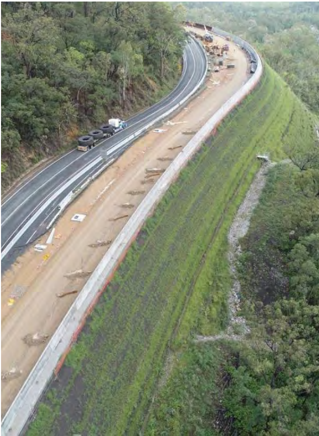
A major construction milestone was reached in late 2018, when works to build the main reinforced earth embankment were completed.
