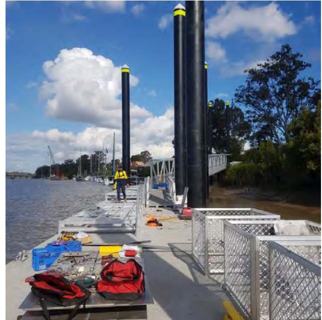
Construction commenced on the March Street jetty in Maryborough.
