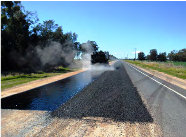
Road resurfacing works on the Cunningham Highway near Goondiwindi.
