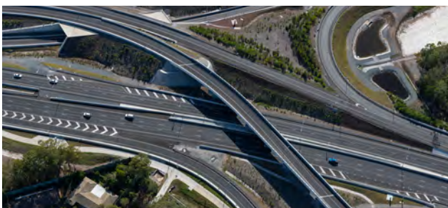
Aerial view of the Deagon Deviation (looking south) on the Gateway Upgrade North.
