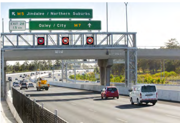
Road operations on the Ipswich Motorway.
