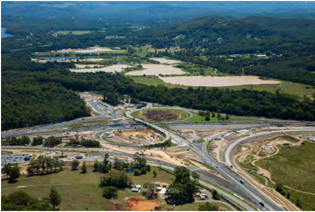
Aerial view of the Caloundra Road interchange.
