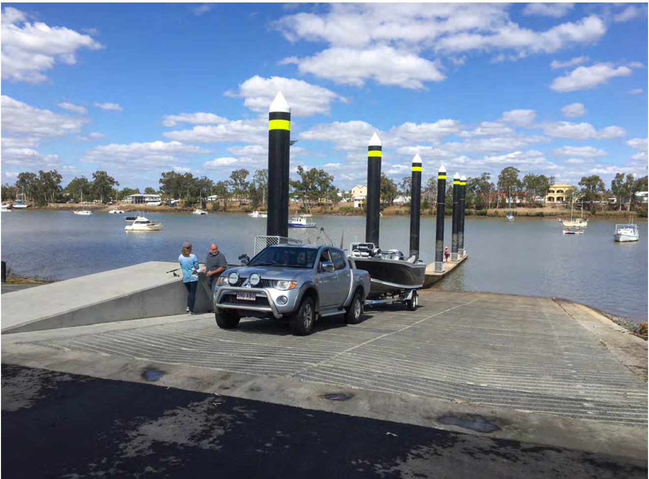
The new four-lane boat ramp at Robert Clark Drive in North Rockhampton.
