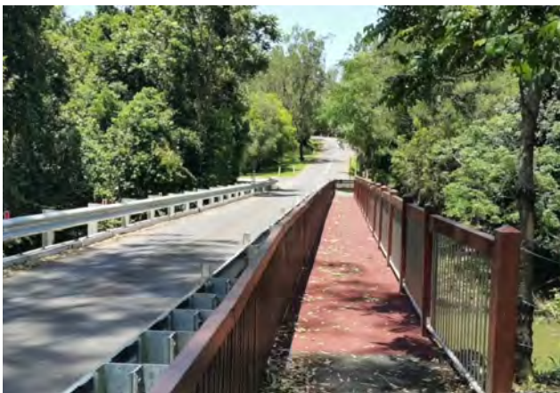
Completed works on the Broken River Bridge including new walkway making it easier for the community to 'spot a platypus'.
