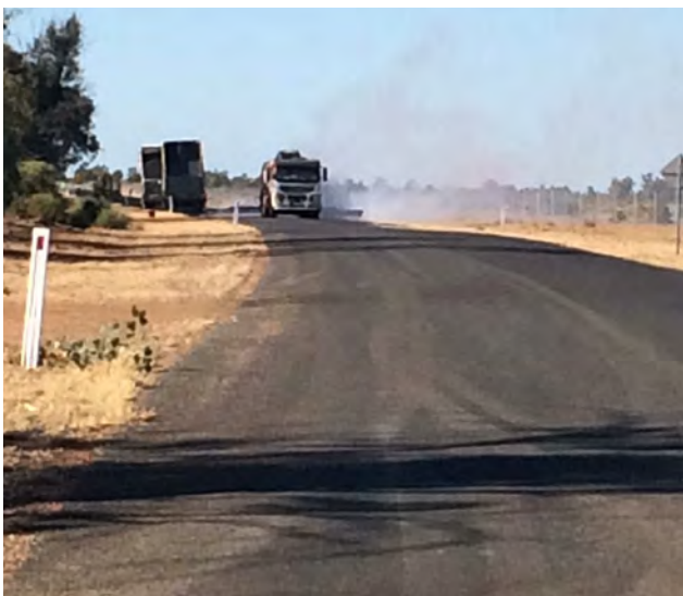
Reseal works on Mitchell-St George Road.
