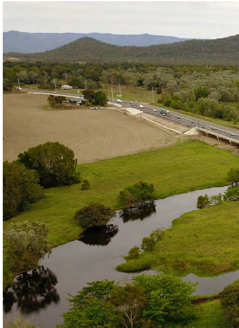
Completed 644 metre long Cattle Creek Bridge, south of Ingham.
