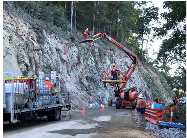
Landslip reconstruction works progressing along Gold Coast-Springbrook Road.
