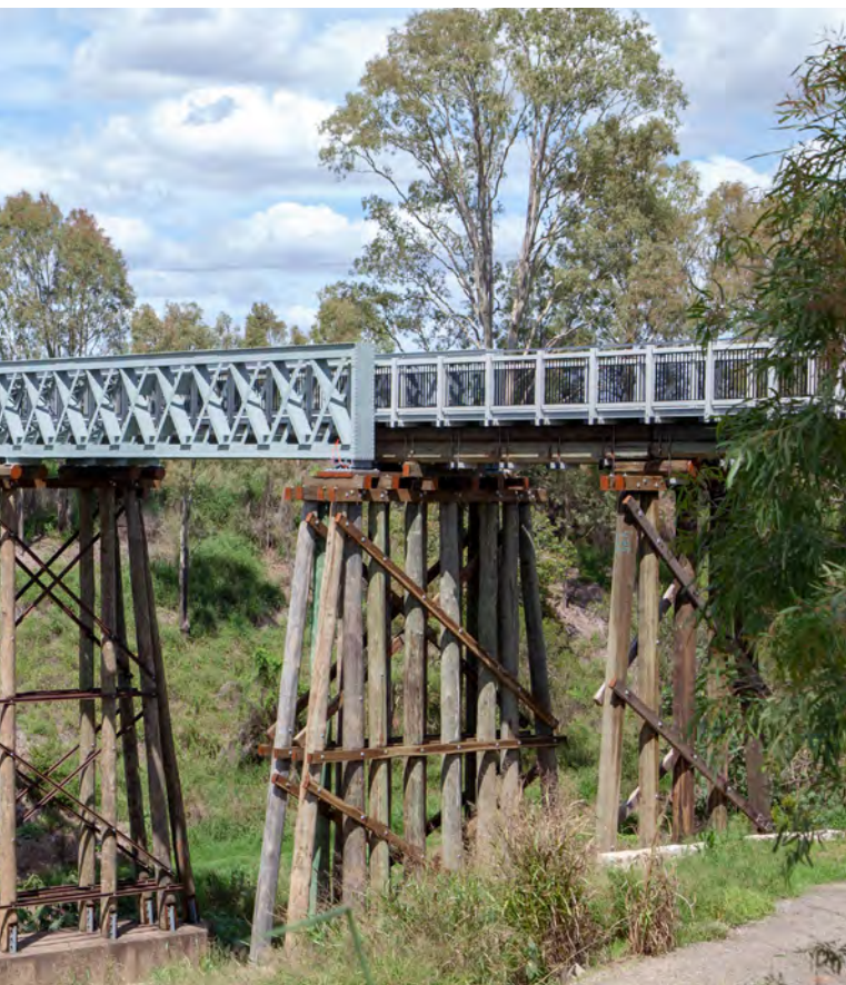
The recently completed heritage listed Lockyer Creek Railway bridge.
