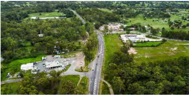
Aerial photo of the Mount Lindesay Highway at North Maclean prior to works starting.
