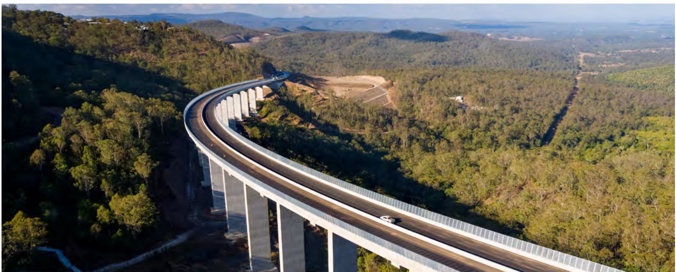
Aerial view of Toowoomba Second Range Crossing.
