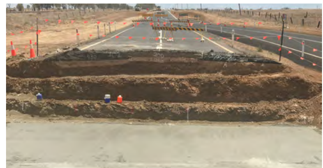
Roadworks on Warrego Highway at Carroll Creek.
