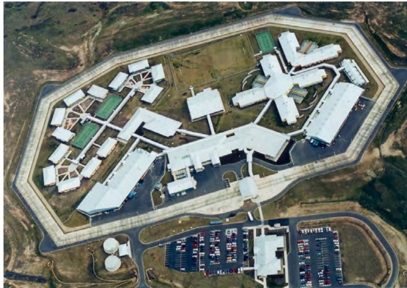
Aerial View - Wolston Correctional Centre
