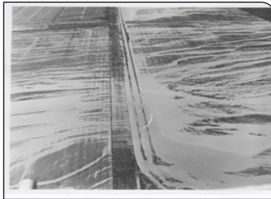
Figure 10.20: Floodwaters spreading across a low level road on the Darling Downs
