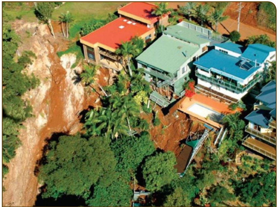
Figure 1.4: A landslip at Currumbin Hill Gold Coast, July 2005 (State of Queensland 2008)
